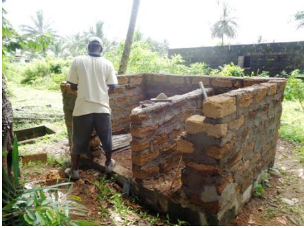
Constructiion of pit latrine for the King's
